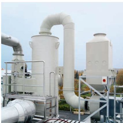
System REITHER scrubber for dust separation in the chemical industry
